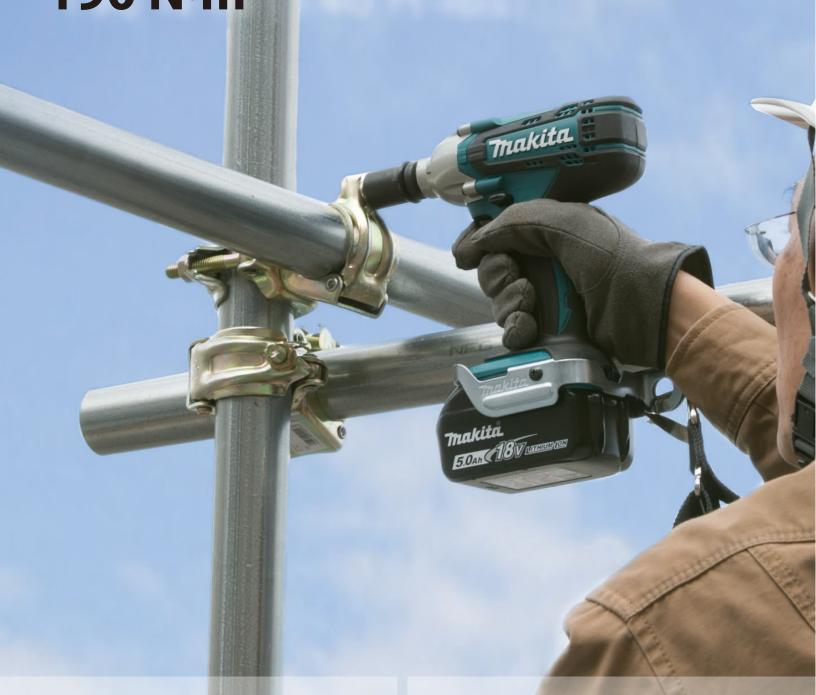
\* Tightening torque at 6 seconds after seating, when tightening M16 (grade 10.9) high strength friction grip bolt.
